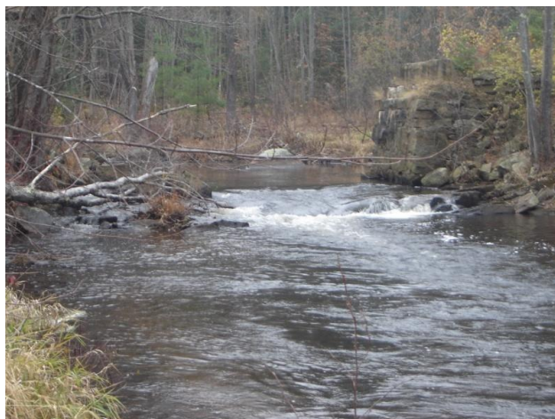
Photograph 7. Remainder of North Waterford Dam, 2011 (J. Pellerin).
