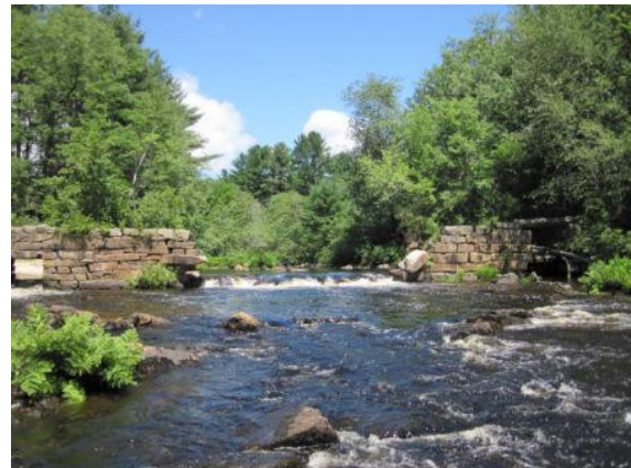
Photograph 4. Remains of Edes Falls Dam around 2005 (MDEP).
